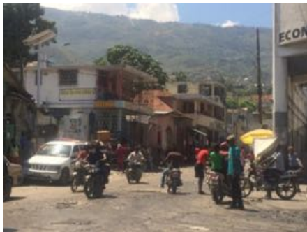
Fig. 1: An uncharacteristically quiet street corner in downtown Port au Prince, Haiti. Solar powered street lights installed under the previous administration are visible, as well as the piecemeal electrical grid wiring, which currently only supplies power between 7pm - 11pm.
