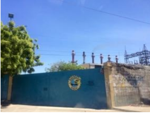
Fig. 2: A typical concrete wall separating the population from costly investments; in this case, the primary diesel generating station of Electricite d’Haiti (EDH)
